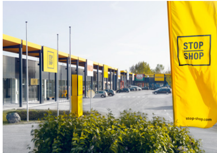
STOP SHOP Simmering Simmering | AT approx. 4,400 sqm of rentable space
